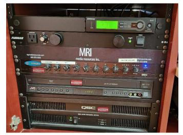
The main power button at the top right needs to be turned on for audio to function.
